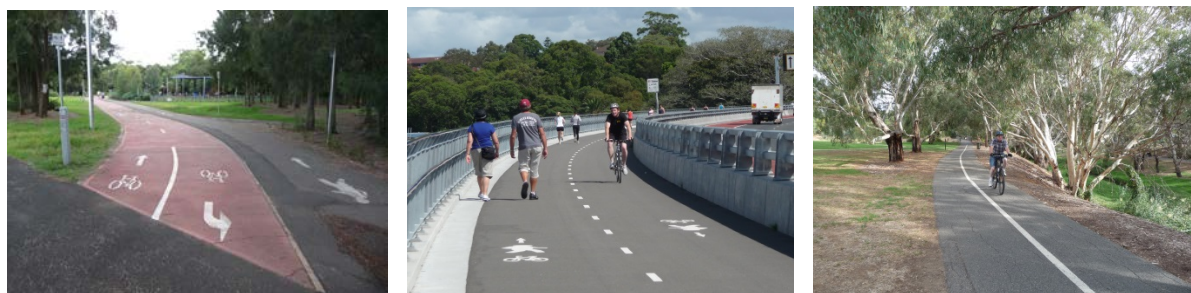
Cycling infrastructure and clear signage is important in supporting the uptake of active transport.
