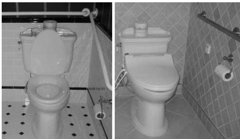
Figure 37: Grab rails in bathrooms
