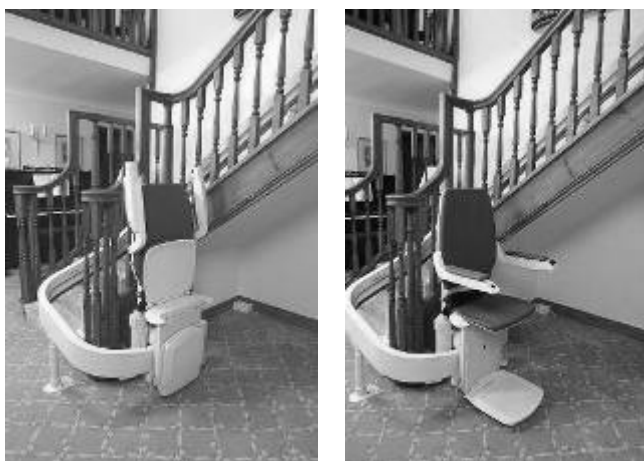
Figure 32: Staircase modified with a stairlift
