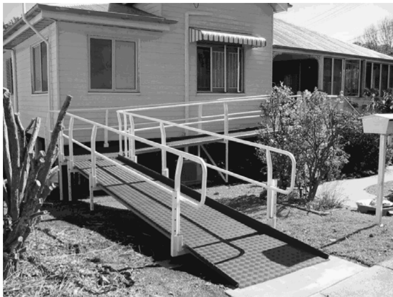
Figure 31: Home modified with a ramp for access
