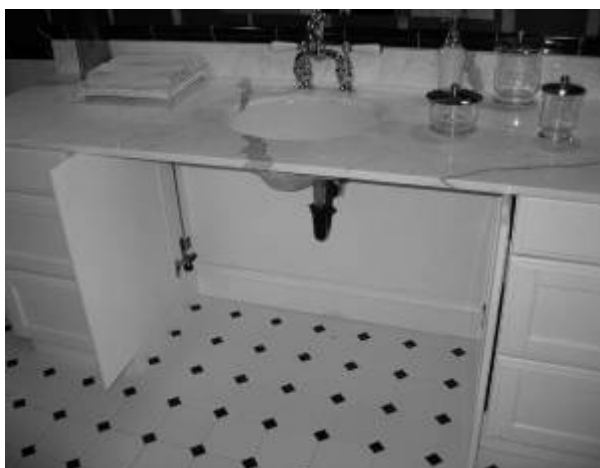
Figure 41: Provision of access without compromising storage
