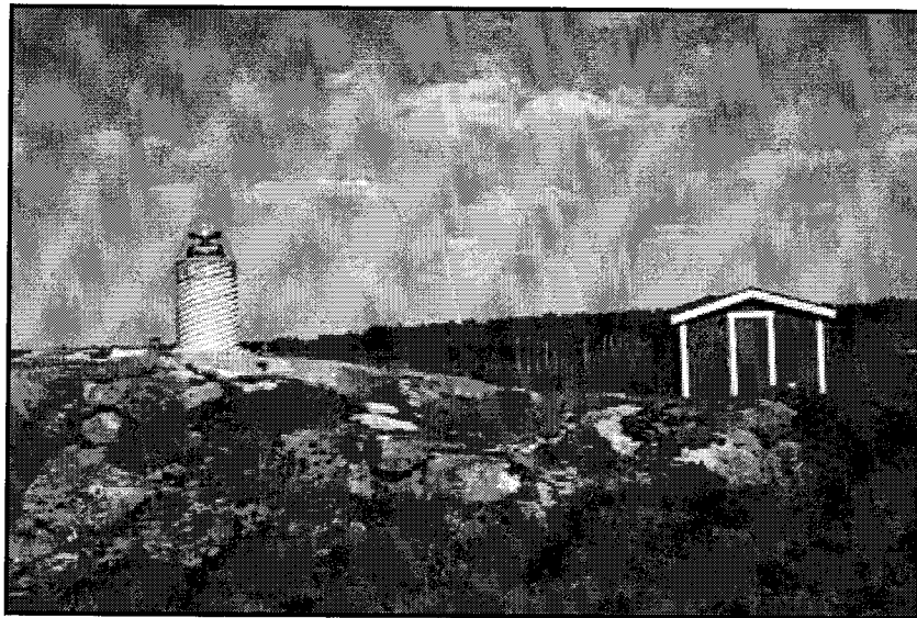
Figure 3.3 - Continuous GPS SWEPOS station Joenkoeping. An example of a very stable, expensive monument (SWEPOS, 2001).
