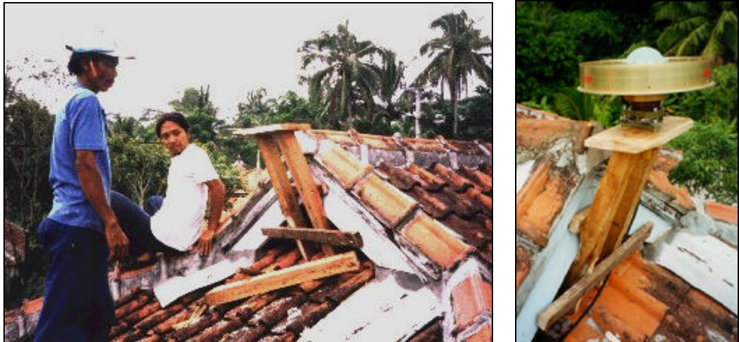
Fig. 2.16: Construction of a GPS antenna platform on the roof of the VSI observatory at Galunggung
