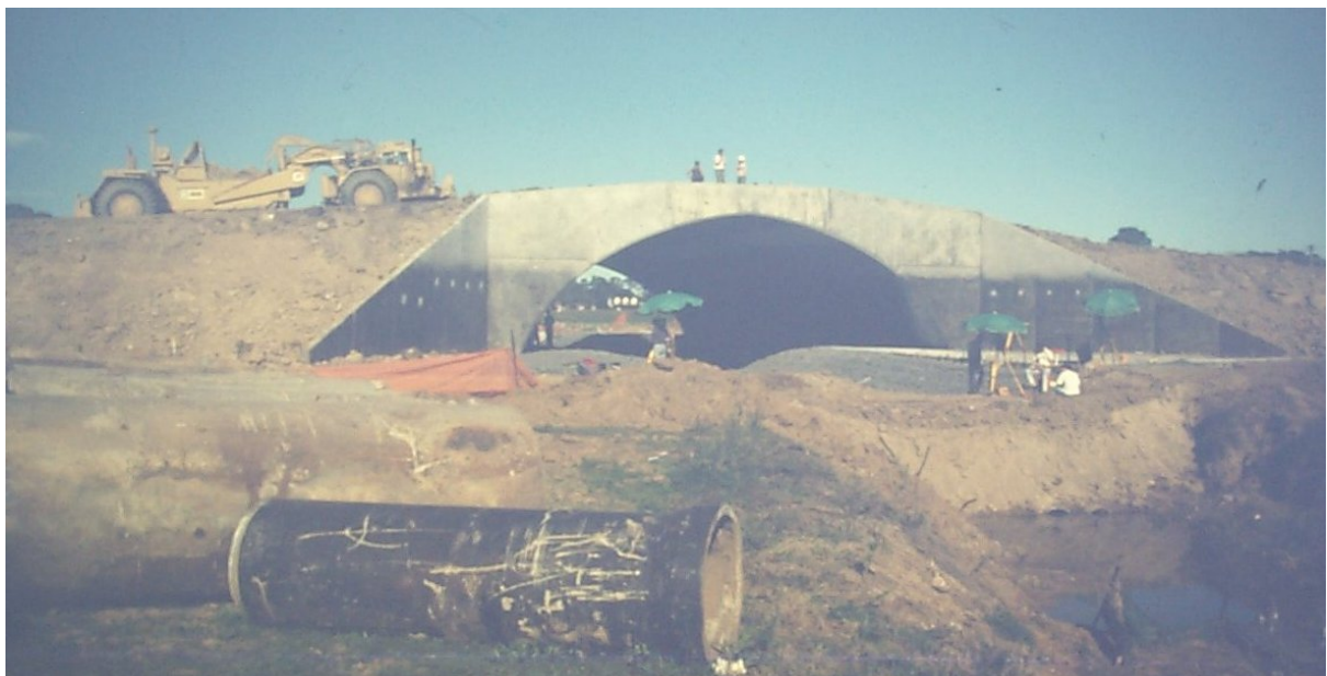
Figure 2 : Surveying during the All-Day Monitoring session. (different photos in actual paper)
