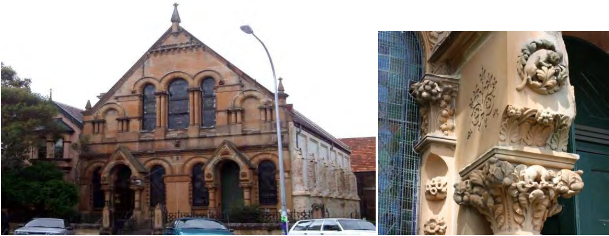
Fig. Façade of the Annandale Creative Arts Centre and a close-up photo of some of the sculptures
