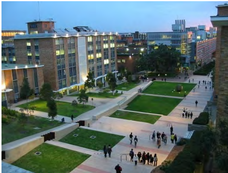
Photo. Mech Eng building with roof top Lightning Conductor pole
