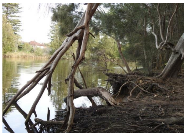
Figure 1 Shoreline erosion of Manly Lagoon, NSW, Australia (Photograph taken 26 th June 2016).
