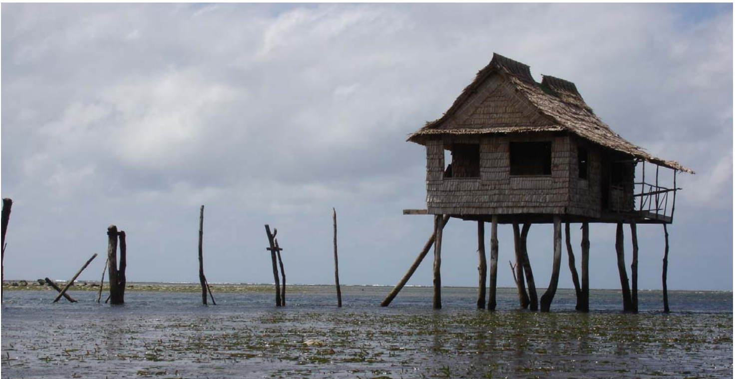
Cyclone damaged building, Solomon Islands
