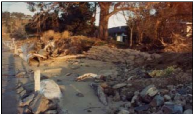
Image 2: Erosion on the end of a rock wall, Roches Beach 2010
