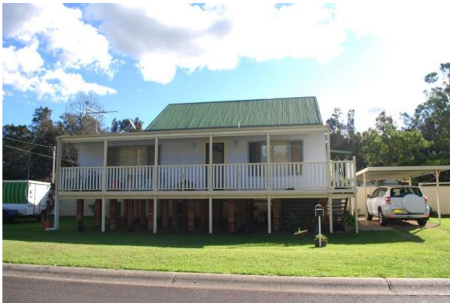
Image 11: Adaptation to increased flood risk – Lake Macquarie City Council, NSW
