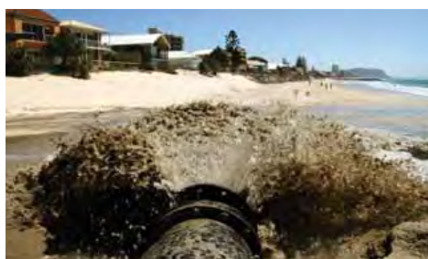
Sand pumping at Palm Beach, Queensland.
