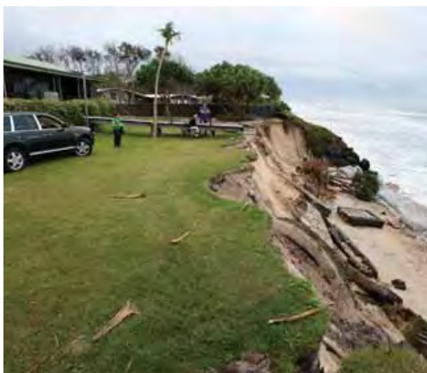
Severe beach erosion along Belongil Beach at Byron Bay, May 2009, where many metres of sand were washed away.
