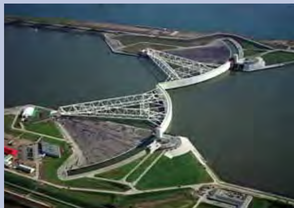
The Maeslant Storm Surge Barrier, The Netherlands.
