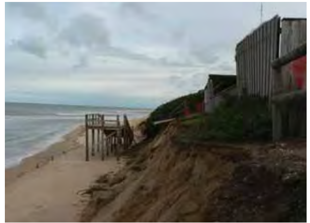
Erosion along Ninety Mile Beach.
