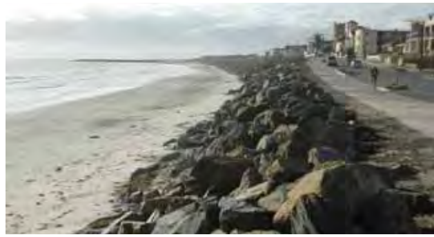
Rock seawall along Adelaide's West Beach.
