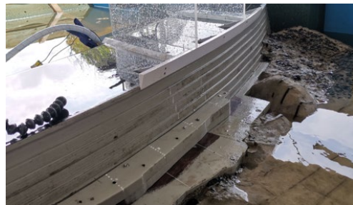
(a) Crown wall and concrete slab removed (partially)
