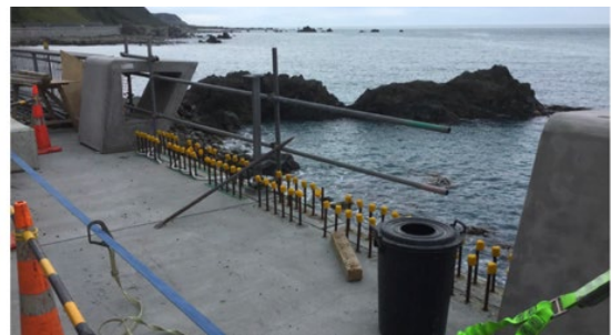
Figure 18 Construction of new crown wall
