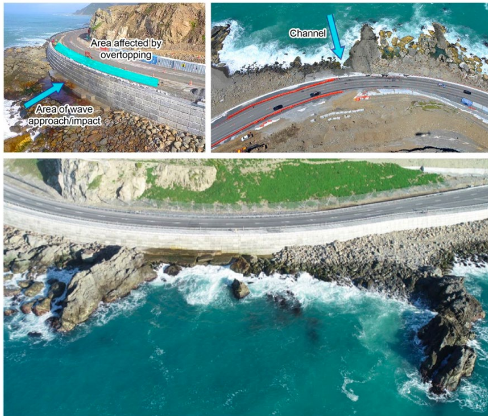
Figure 3 Overview of Ōhau Point post-rehabilitation works [Source: NCTIR]
