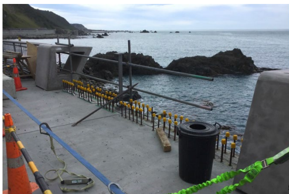
Figure 13 Installation of a crown wall at Ohau Point
