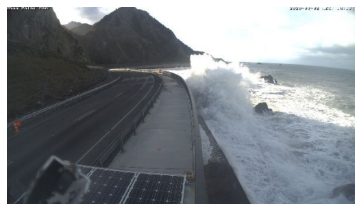
Figure 12 Example of low level overtopping identified at 2pm on 2/7/20
