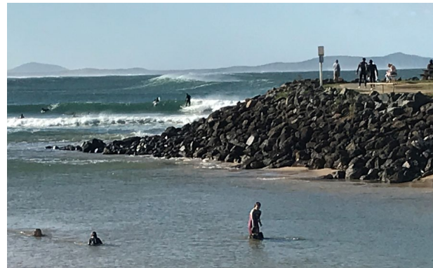
Figure 6 Angular and rounded rock enhancement of existing cobble foreshore at Crescent Head NSW. Note adjacent surf break (James Carley)
