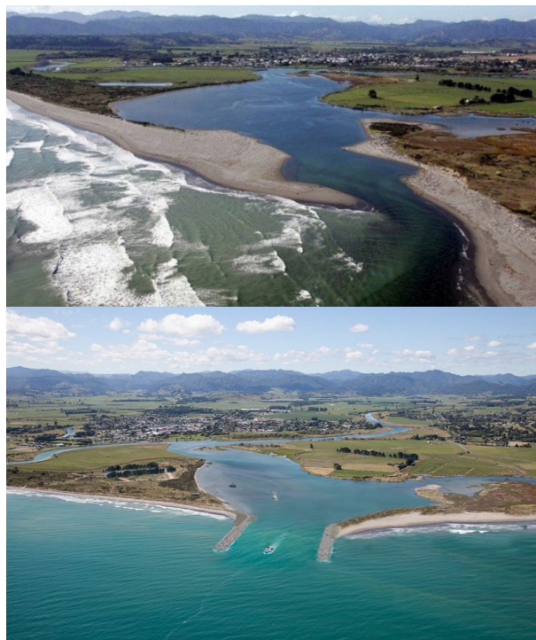
Figure 1: Existing Waioeka River entrance and proposed including river training works (source: ODC|stuff.co.nz)
