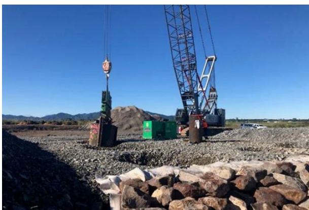
Figure 5: A DC trial was conducted on site to assess the likely depth of improvement and potential damage to geotextiles.
