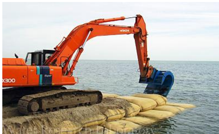
Figure 2.20: Placement of Smaller Geotextile Bags by Special Excavator Bucket
