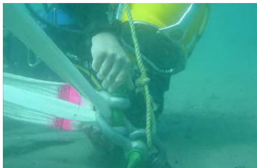
Securing Reef Panel to Seabed Anchor
