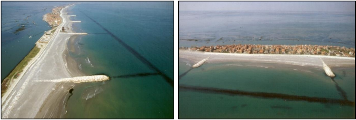
Figure 4.4: Successful Submerged Breakwater, Pellestrina Island in the Venice Lagoon, Italy (in conjunction with groynes) (Source www.venicethefuture.com )
