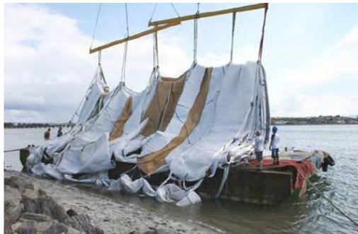
Loading Reef Panel onto Barge
