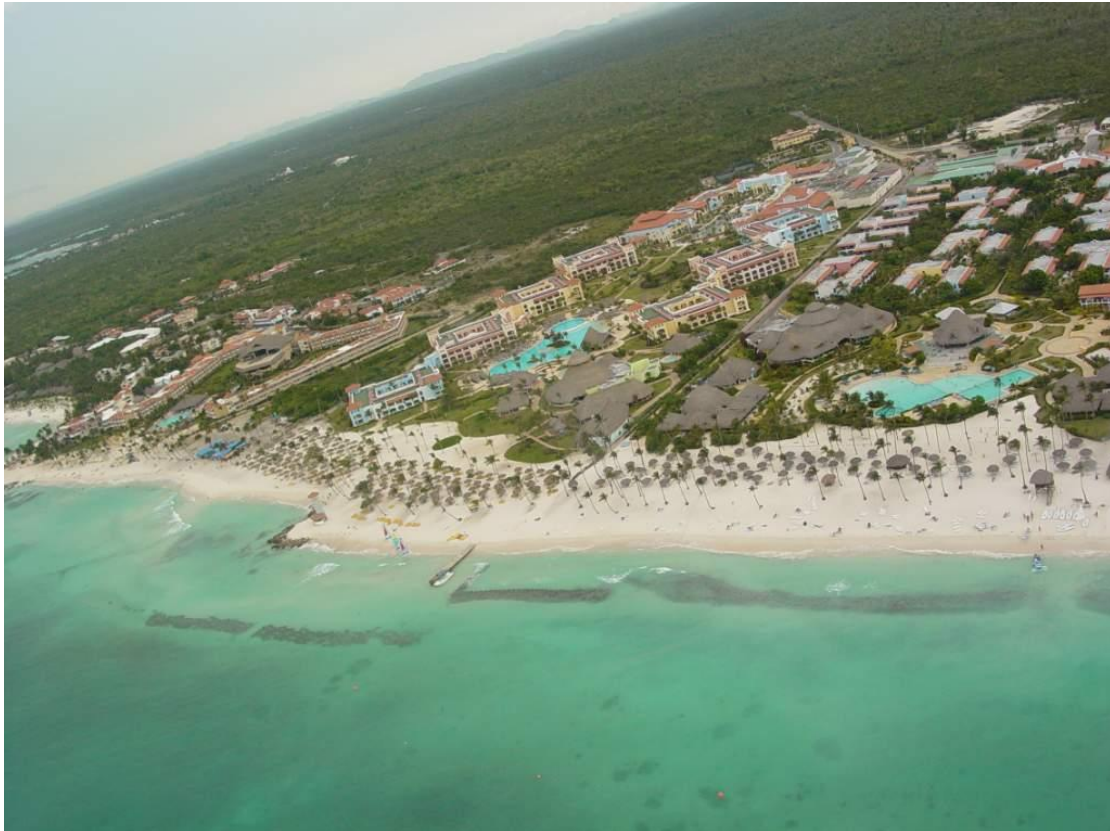
Figure 4.2: Reefball™ Submerged Breakwaters, Gran Dominicus, Dominican Republic (Source: www.reefball.org )
