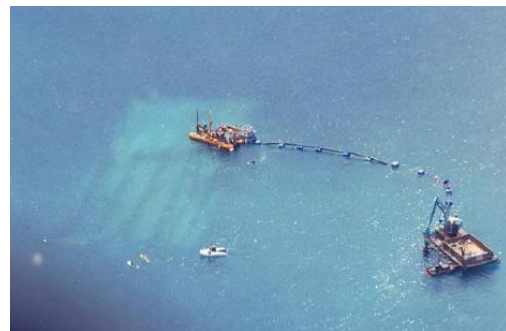
Filling Geotextile Tubes
