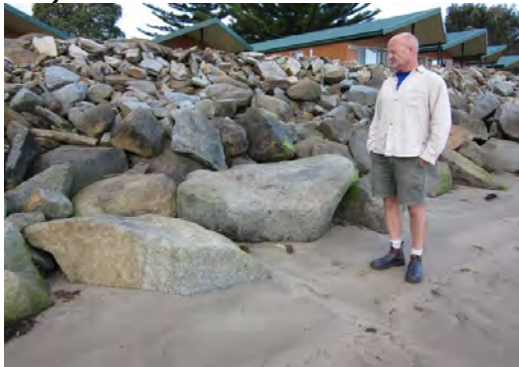
c) Rock wall armour properties are mixed
