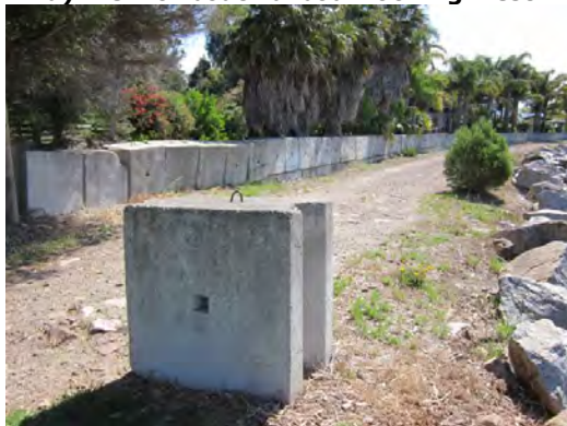
c) Concrete cube wall seaward of development
