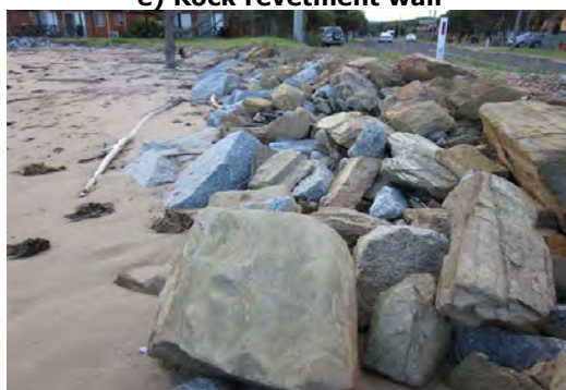
g) Rock wall armour properties are mixed
