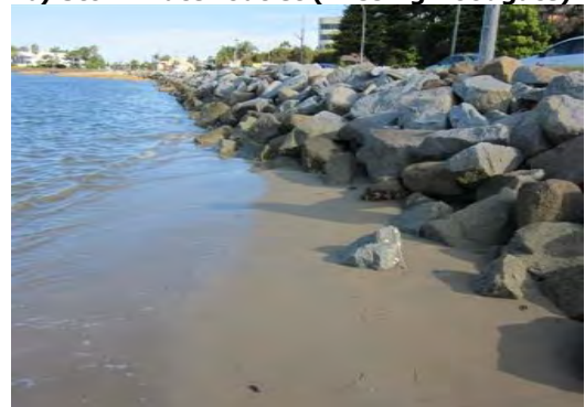
d) Revetment rock armour type 2 of 2
