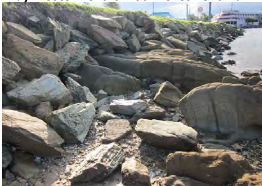
c) Revetment rock armour type 1 of 2
