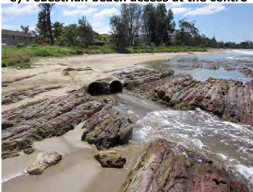
g) Stormwater outlet at southern end
