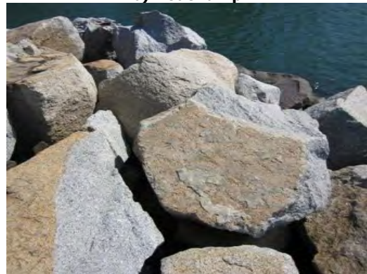
d) Typical primary rock armour
