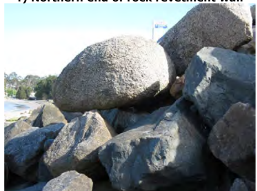
h) Example of precariously positioned rock
