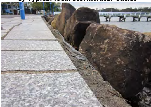
g) Geotextile underlayer visible
