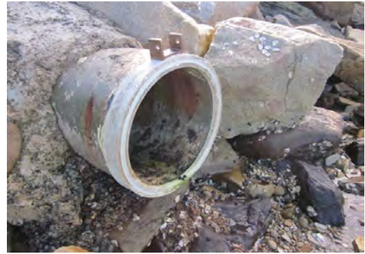
b) Stormwater outlet (missing floodgate)
