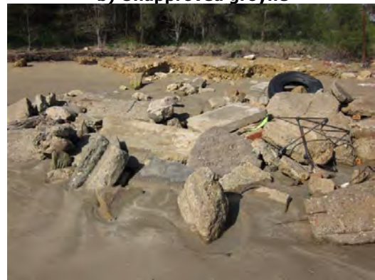
d) Building waste used as groyne armour
