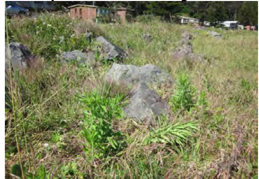
d) Partially buried rock revetment wall
