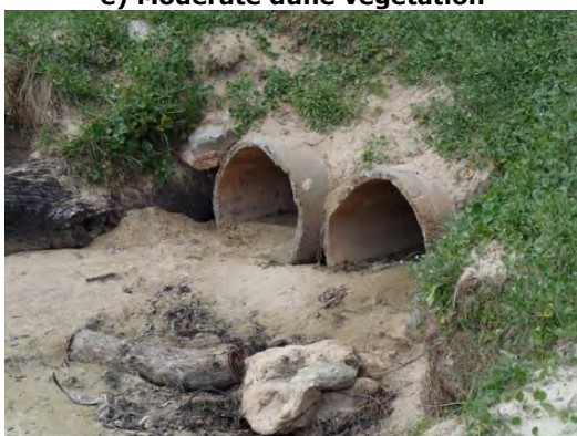
g) Stormwater outlets at the southern end
