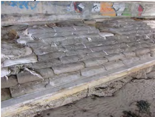
c) Scour protection at bridge abutments
