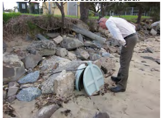
f) Stormwater outlet (blocked floodgate)
