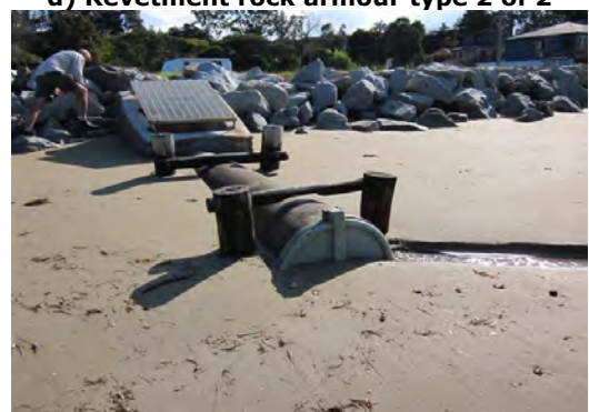
f) Stormwater outlet (blocked floodgate)
