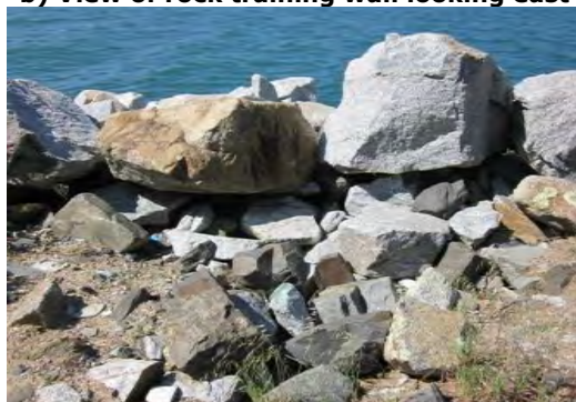
g) Typical secondary rock armour
