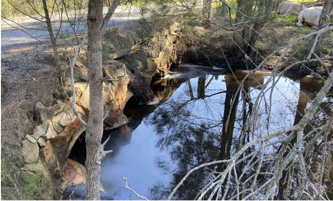
Figure 2-3: Culverts beneath Springbank Rd (Photo: Shoalhaven City Council)
