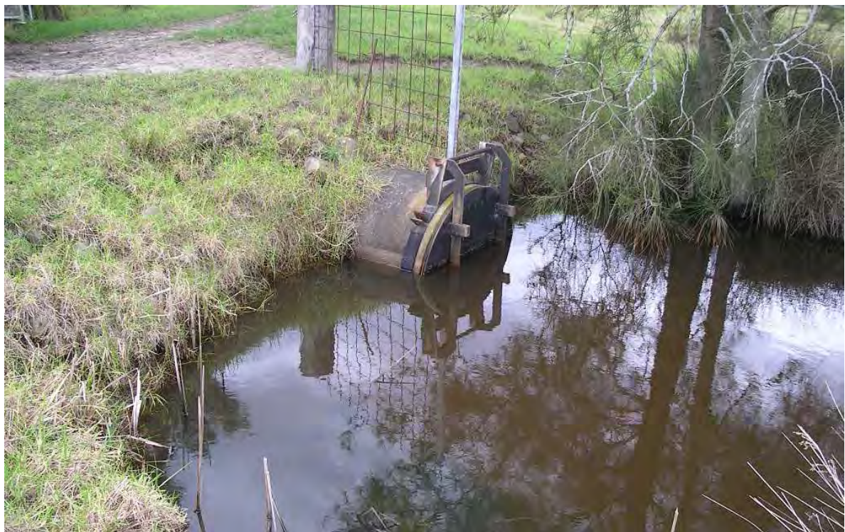
Figure 2-4: Private structure on side drain (Photo: S. Nichols/DPI)
