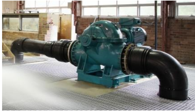
Figure A-1 Brook Crompton centrifugal pump
