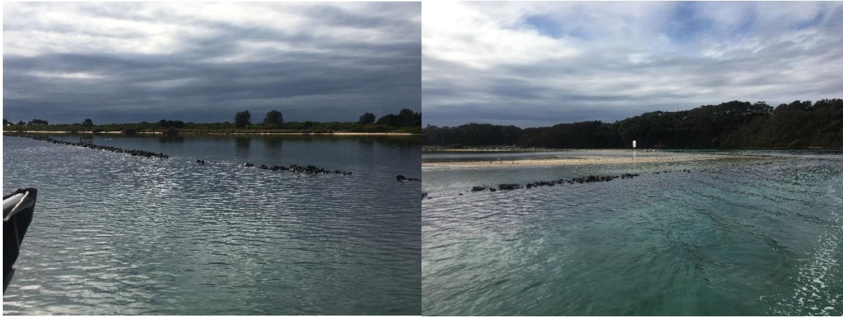
Figure 3-8 Breakwater weir crest estimate using main channel water level
