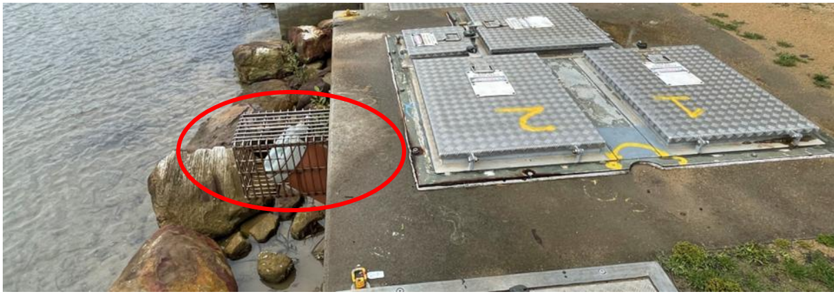
Figure 2-1 Example of a sewage pumping station overflow point (Careel Bay, Pittwater)
