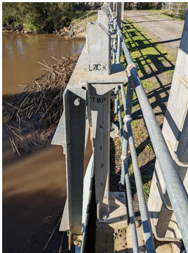
Figure B.3 The lifting mechanism on one of the floodgate flaps
