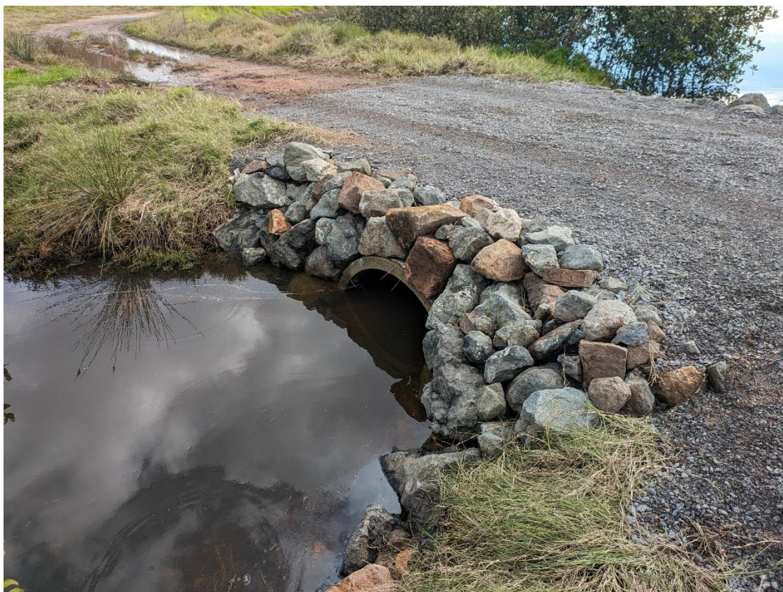
Figure B.12 A 0.9m diameter culvert underneath Hartin's Track allowing Hartin's Creek to flow
