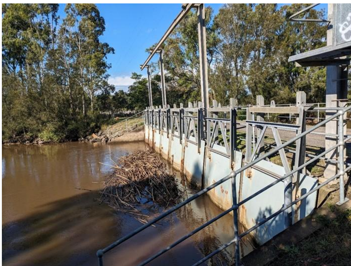
Figure A.12 Ironbark Creek floodgates with gates lifted to maximum opening height
