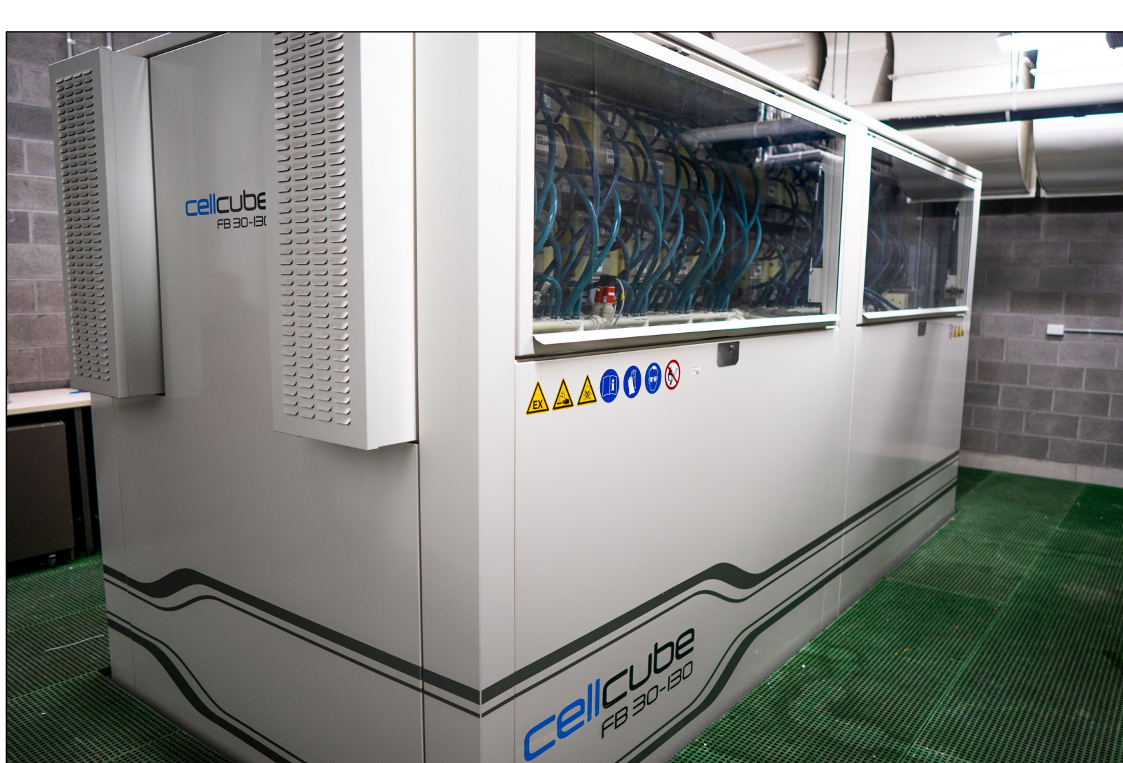
30kW/130kWh Vanadium Redox Flow Battery installed at the UNSW Tyree Energy Technologies Building
