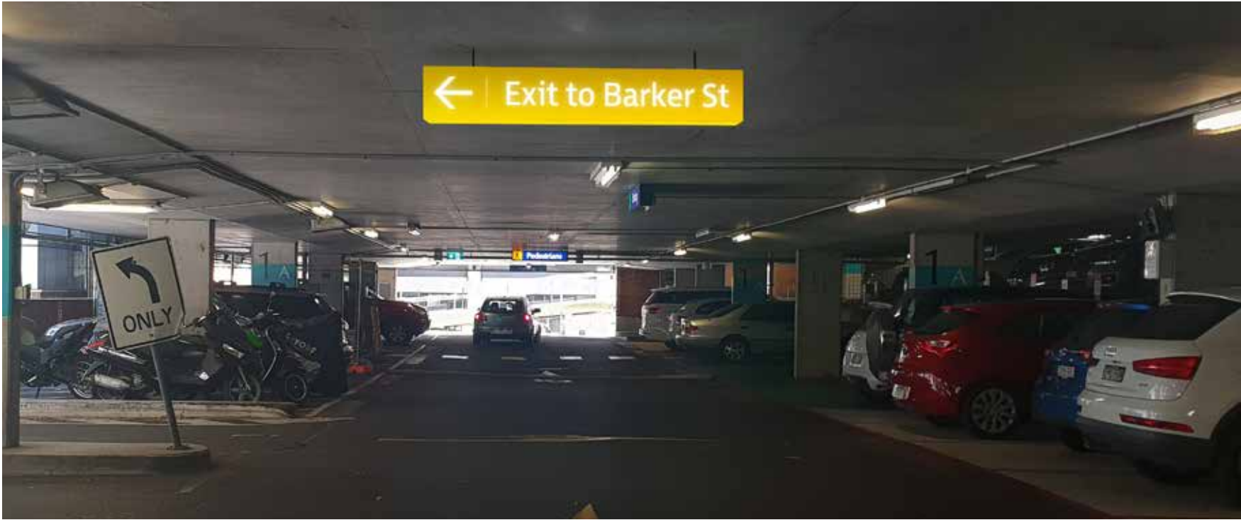
01 Car Park Suspended Directional Baker Street Parking
