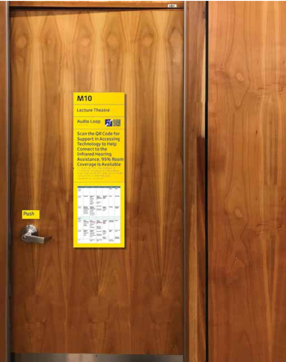
01 Room ID Lecture theatre configuration (obstruction on door hardware side so positioned direct to door)
