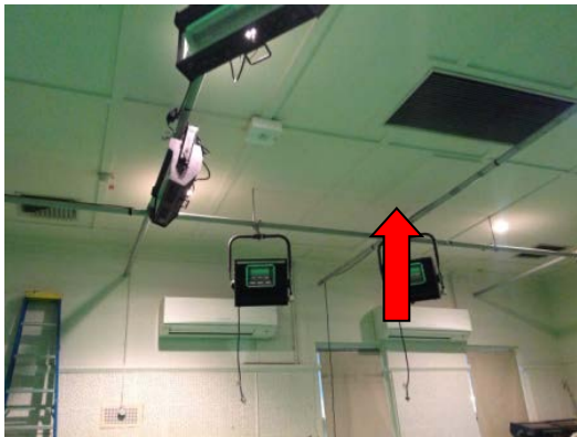
Figure 3: COFA Campus, Block C, Ground Level, Room CG11, Ceiling – Fibre Cement Sheeting
