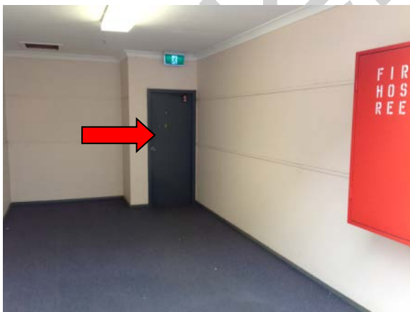
Figure 11: Randwick Campus, Building R9 Tram Shed, Mezzanine Level, Room MQ2, Stairwell – fire door core
