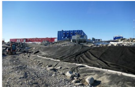
Figure 2. Casey station where bioremediation of fuel spills is ongoing using engineered biopiles combined with nutrient amendment.
