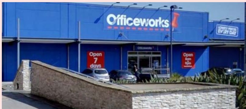
Fig. A2. Front view of the building.
