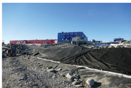
Figure 2. Case station where bioremediation of fuel spills is ongoing using engineered biopiles combined with nutrient amendment.
