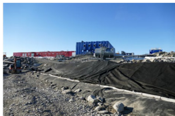
Figure 2. Casey station where bioremediation of fuel spills is ongoing using engineered biopiles combined with nutrient amendment.
